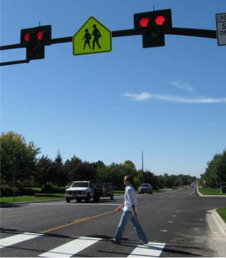
Figure 11 – Pedestrian Hybrid Beacon (PHB)
