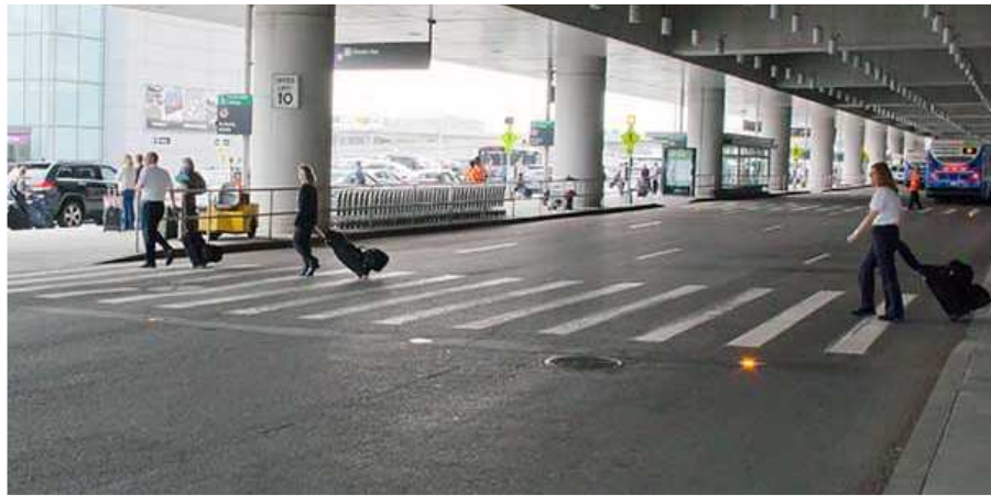
Figure 12 – In-Road Pedestrian Lights
